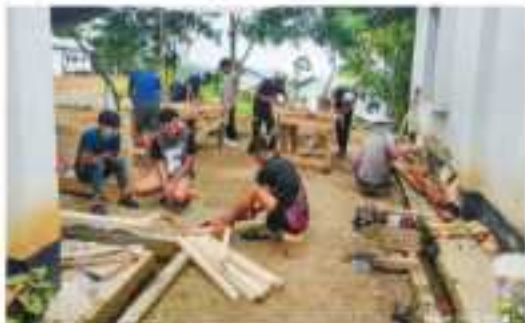
B-109 Carpenter Practice
